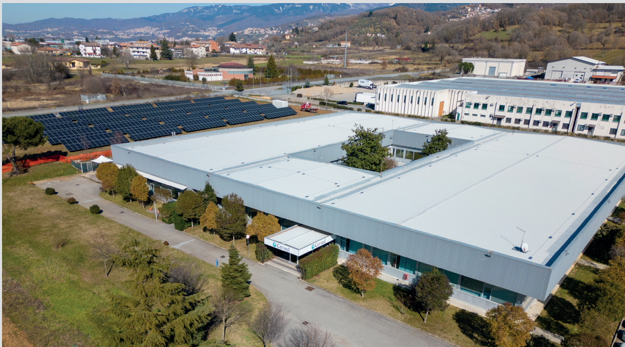
Photovoltaic system installed at the Mangone (CS) site
